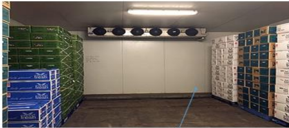
Cold storage Area
